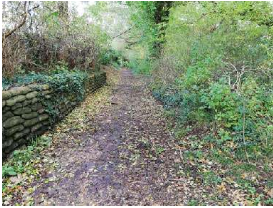
Former rail line parallel to Fairlee Road
