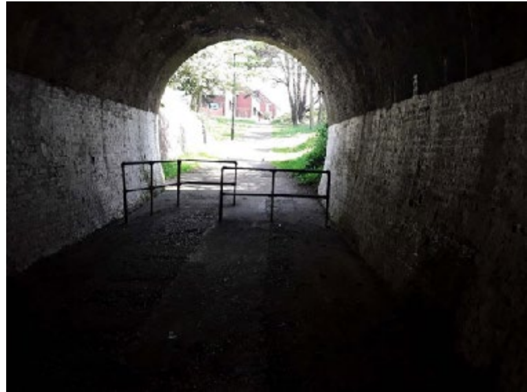
Tunnel under Fairlee Road
