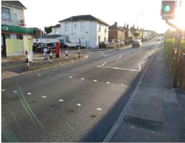
Junction of Binstead Hill and Chapel Road
